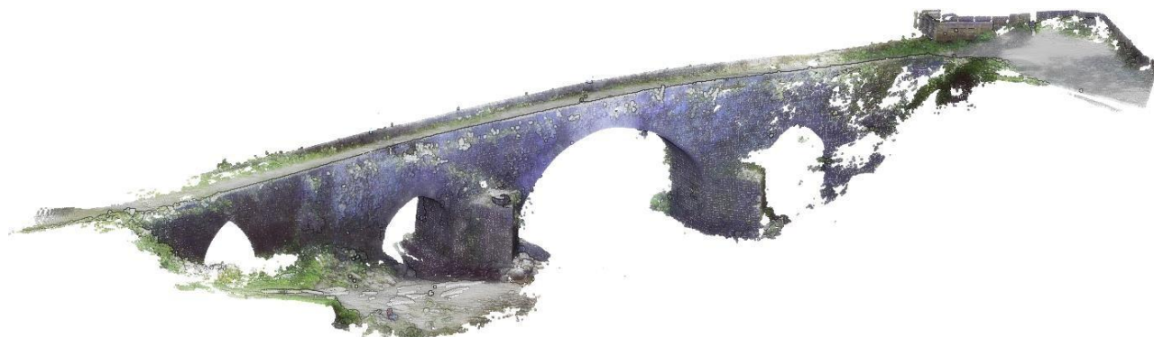
Fig. 4. Point cloud of the bridge cleared of surrounding vegetation and noise.
