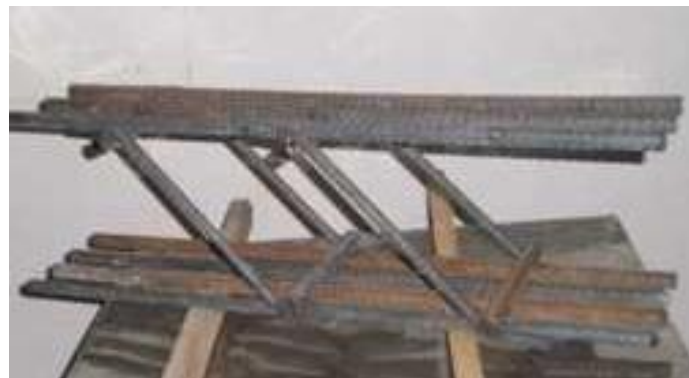
Fig. 1: Typical welded swimmer bars
